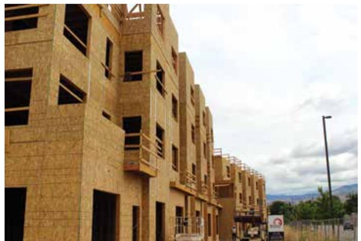
*7/16 inch OSB wall sheathing wraps the structure.*
