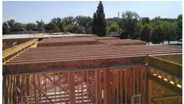
*I-joists between the first and second floors. Courtesy of Steed Construction.*
