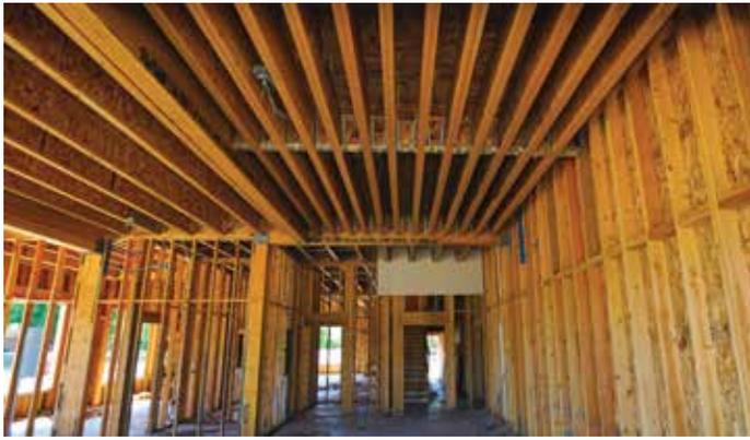
Laminated veneer lumber joists at 16 inches on-center support three stories of bearing walls above.
