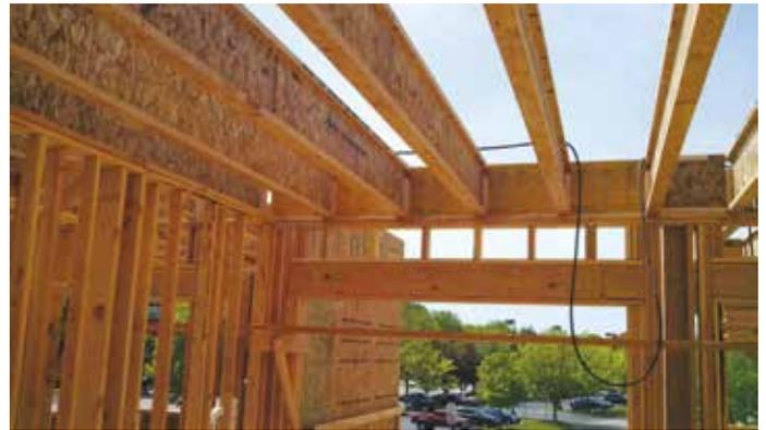
*I-joists bearing at an exterior wall and a laminated veneer lumber header over a window opening.*
