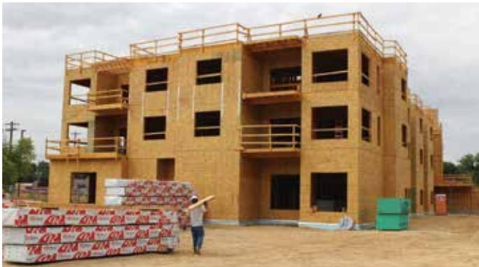
Engineered wood packages are delivered to the jobsite based on the construction schedule.
